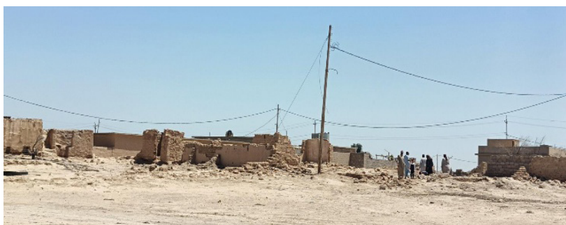
Figure 2 the damage of houses
